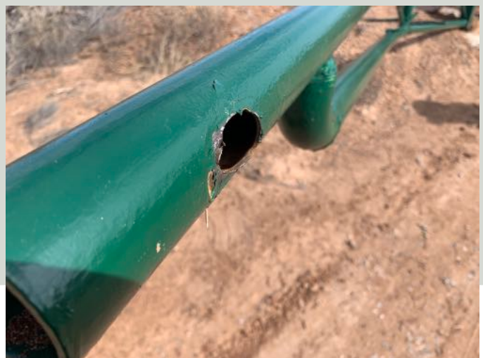
Where the Locking device was welded to the Gate
