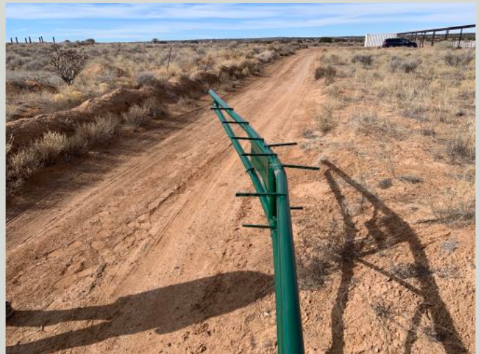
Looks like a Wench was used to pull the gate inward
